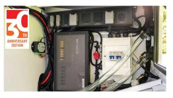
machines your energy savings can be exponential over a 12V system. With the higher voltage and lower amps there is a remarkable saving in voltage drop over distances once again increasing efficiency.
